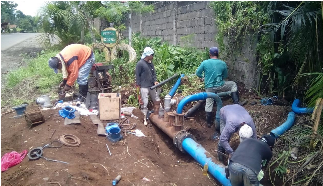
Rehabilitation and upsizing from 6"Ø to 8"Ø transmission pipelines at Damilag, Manolo Fortich
