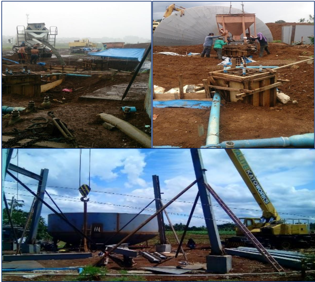
↑ Construction of the 300cu.m. elevated steel tank at Bayabason Extension Project at Sitio Kitam-is and Cebukawan of Brgy. Lonucan ↓
